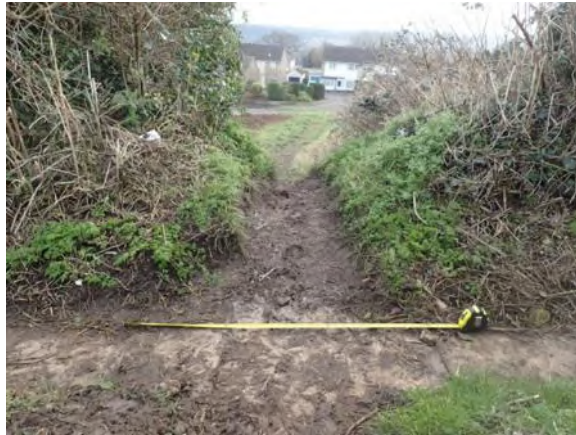
Before: People walking across the ditch had worn away the embankment leading to water spilling towards roads and homes.
