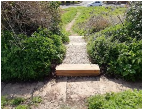
After: Railway sleepers were used to reinstate the ditch whilst also allowing people to access the public right of way.
