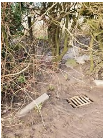
Before: Large amount of silt build up due to inefficient drainage.
