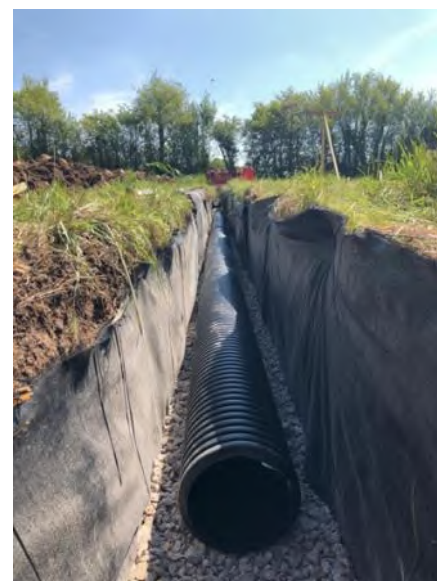
New pipe laid across field to receiving ditch
