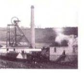
Somerset Coalfield, with a depth of 1,791ft. in 1886. A full range of buildings including a 120ft high chimney, boiler house, winding engine house, offices, saw pit shed, carpenters shop, smith's shop and workers cottages stood on this site known as 'Ham'. The 1905 engine winding house of Middle Pit remains, as does the former Radstock Gasworks building, built by the Waldegrave Estates in 1858 and closed in 1954. The chimney base can also be seen on the left walking up the road.
