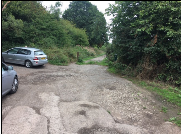
Fig. 1: Point A looking towards gate at point B
