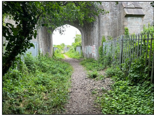
Fig. 2: Point B looking NE under railway
