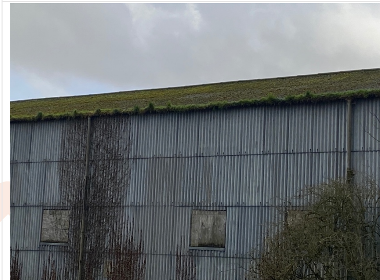
Typical view of roof
