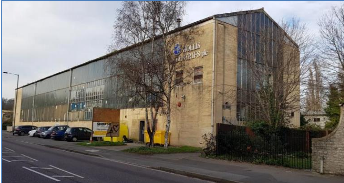
Fig 6. Photograph of the subject building – constructed in 1970. A recent inspection undertaken by CSquared has confirmed that the building has reached the end of its economic life and that for the site to remain in beneficial use the site will need to be comprehensively redeveloped.
