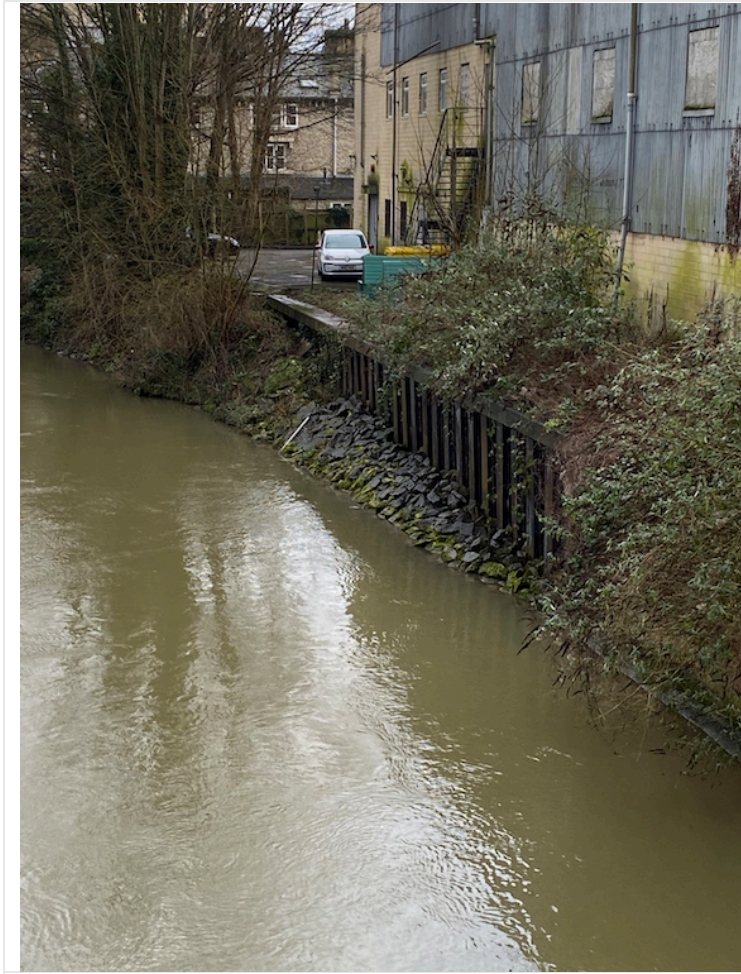
Proximity of north elevation to the river
