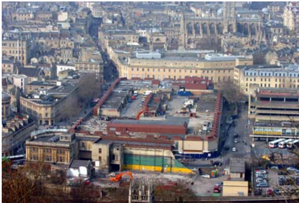
Demolition underway in February 2007
