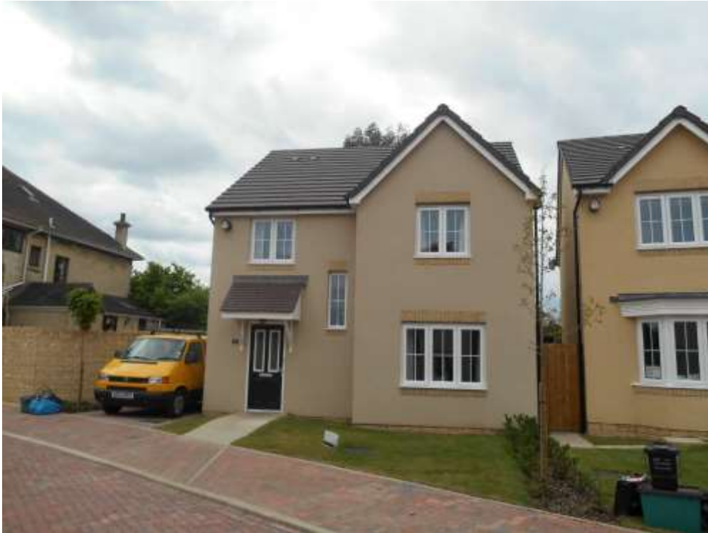
Figure 9 - Low kerbs and lack of steps to property allow easy access for all. Gate to garden on right of image provides route to external storage. Private and public spaces separated with the use of landscaping.
