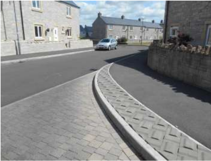
Figure 13 - Traffic calming measures put in place to sharpen the bend and slow traffic.
