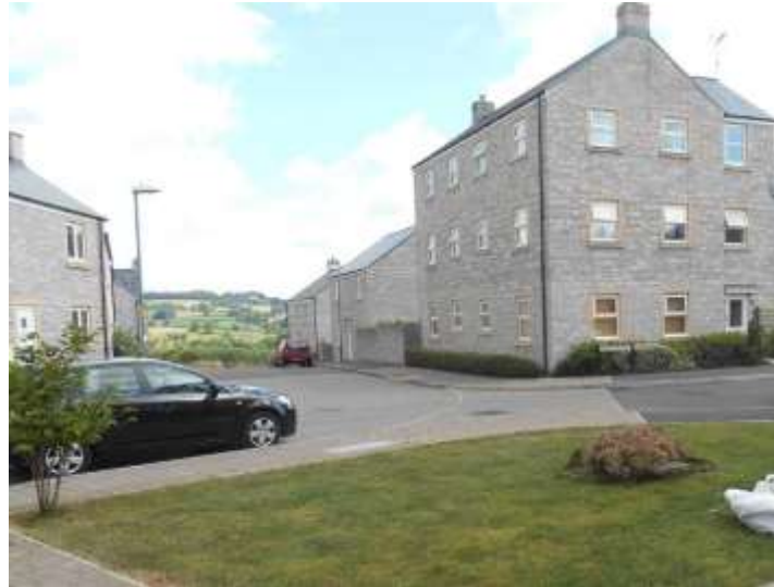
Figure 8 - View of the Mendips through the properties.
