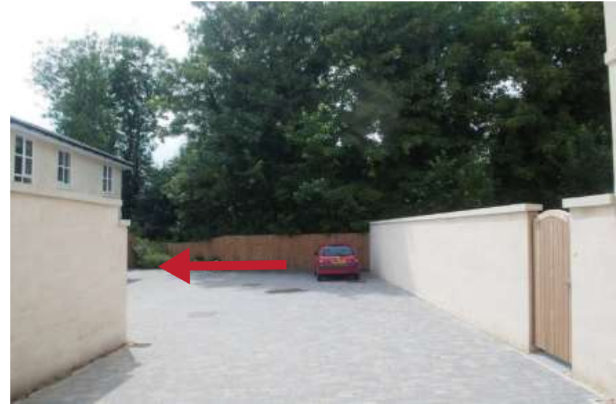
Figure 6. The scheme suffers from awkward placement of front doors in some of units, creating unfavourable thresholds.
