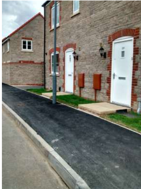
Figure 15. Raised kerbs and change in surface treatment helps distinguish between the different routes and define streets.
