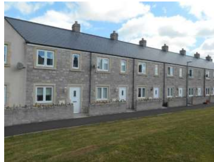
Figure 5 - Terraced housing in development.
