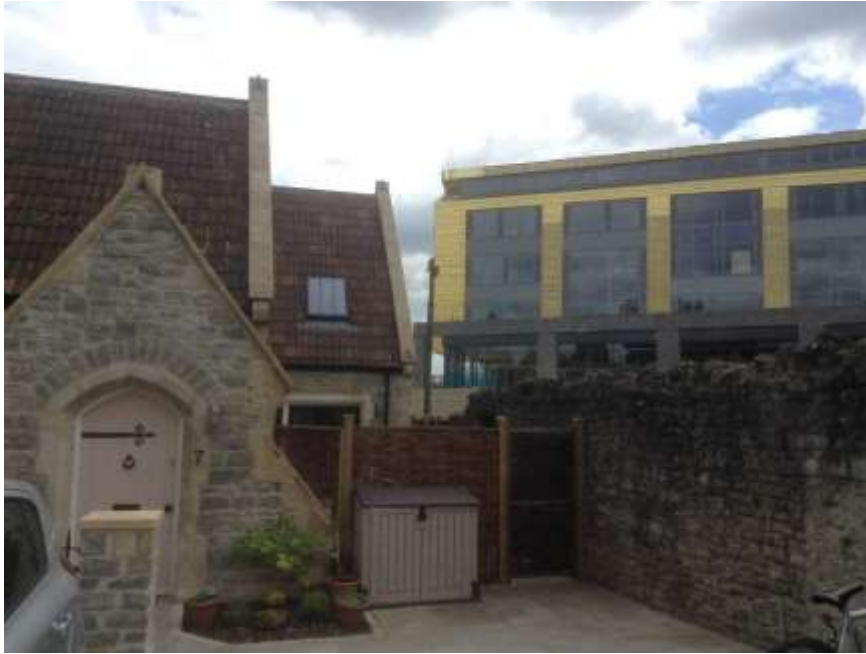
Figure 6. Old school wall has been retained and soft screens have been erected in areas to address issues of privacy. Tasteful landscaping and Fences have been used to distinguish between public and private areas.
