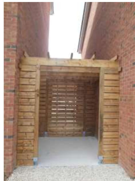
Figure 12 - Waste storage facilities for semi-detached houses.
