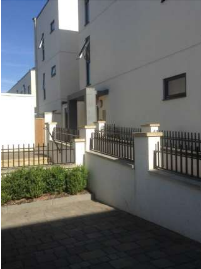
Figure 23. Ramped access at the back of dwelling on Stothert Avenue.
