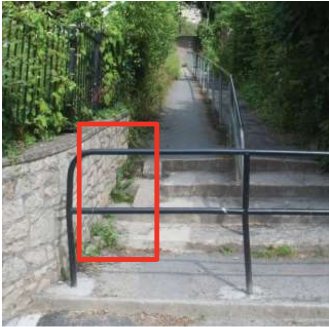
Figure 4. Missed opportunity to contribute positively to local infrastructure by failing to add side ramps for cyclists and improving the footpath.
