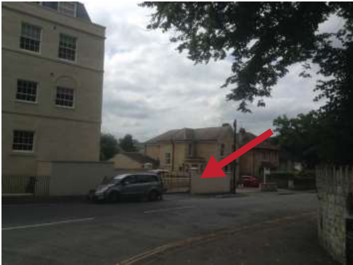
Figure 1. Vehicle access is off the substantially less busy approach to the site.
