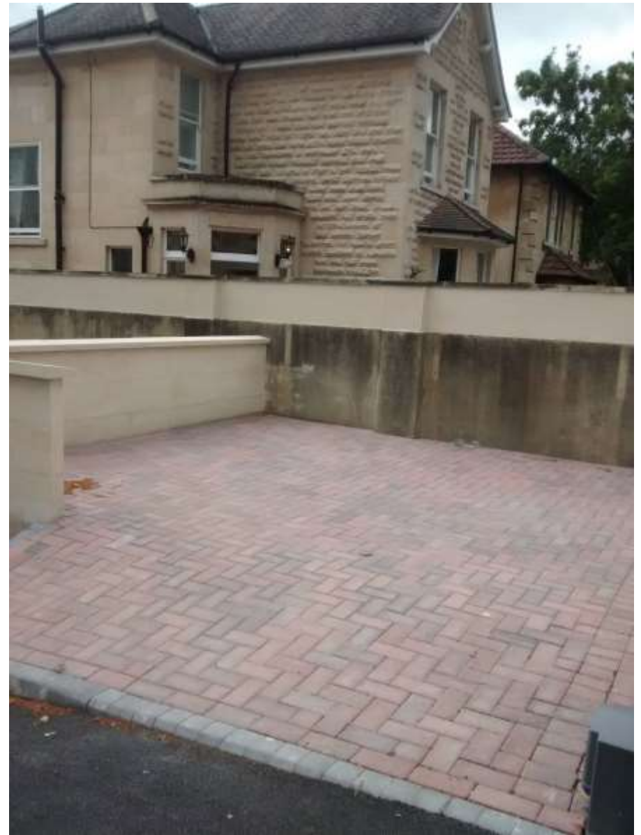
Figure 16. External bins and rubbish storage.
