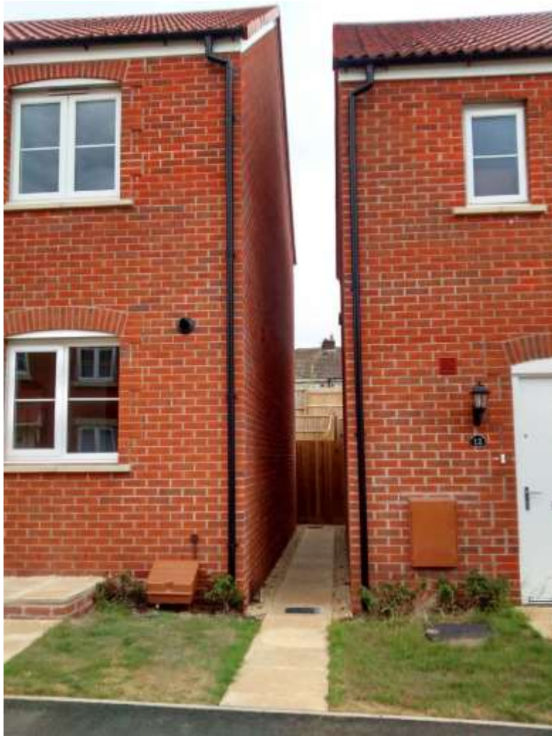
Figure 30. Gaps between semi-detached houses have been used to provide direct access route between back gardens and the front pavements. This will enable ease of movement of rubbish on collection days.
