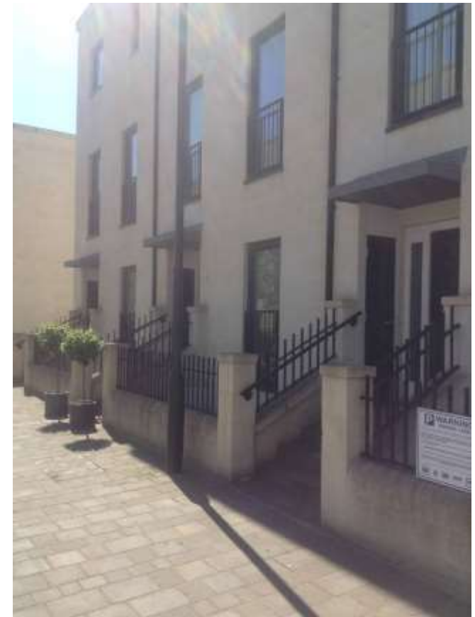
Figure 22. External porch storage
