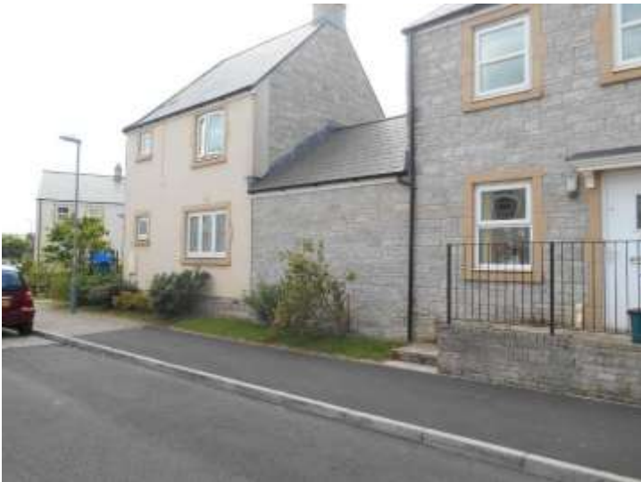
Figure 7 - Examples of building materials used - brick work and render
