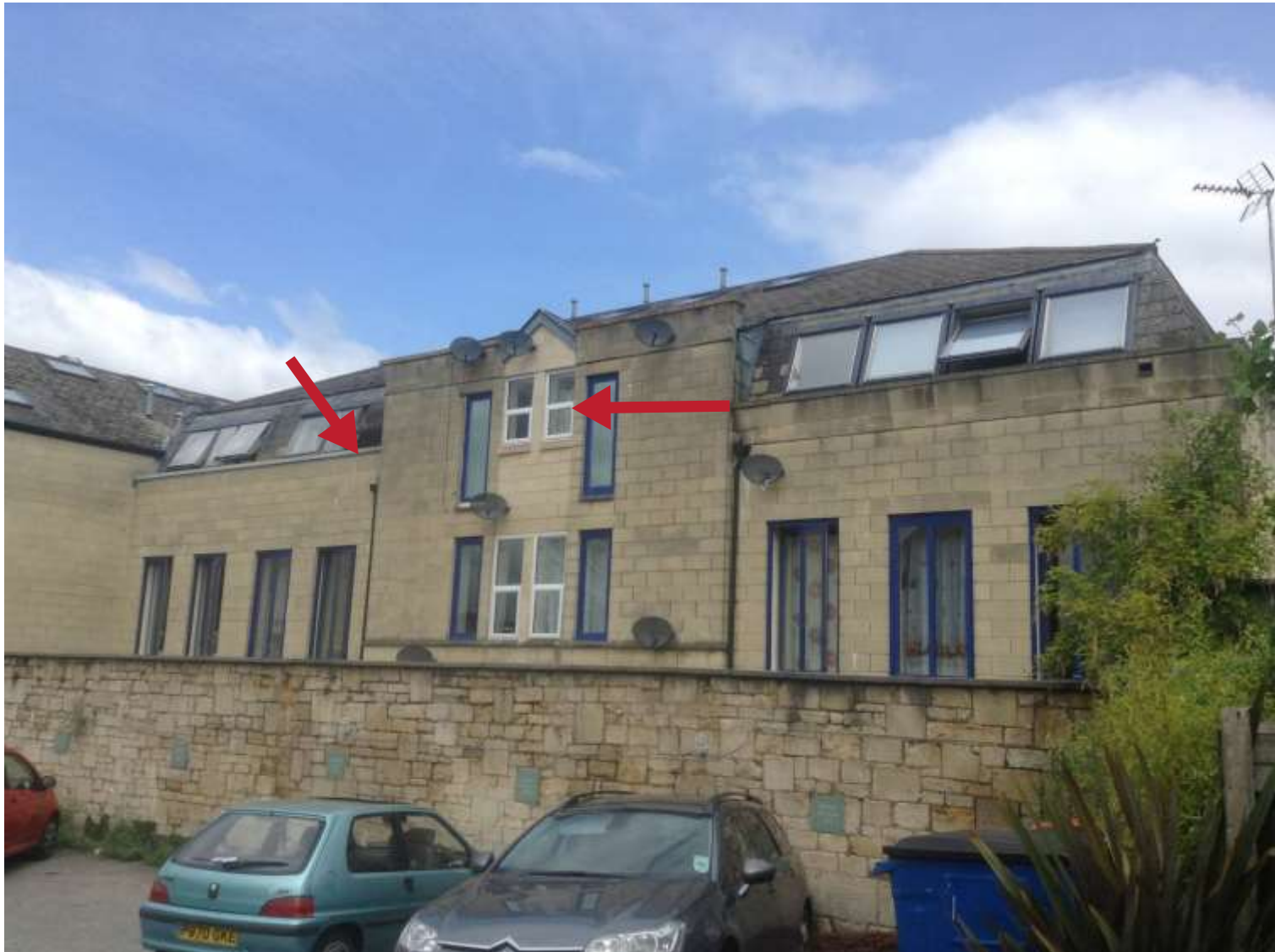
Figure 3. Rear view facade. Image taken from the Bear Pub car par.
