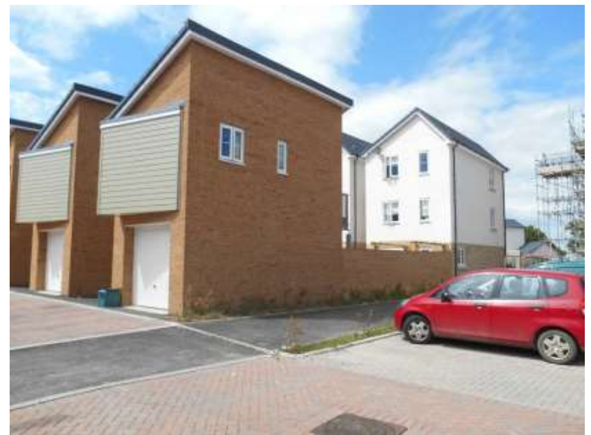
Figure 10 -- Car parking spaces are clearly defined by different coloured brick work.
