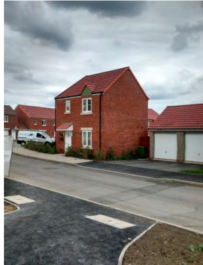
Figure 19. Good level of natural surveillance is provided by windows unto share parking area.
