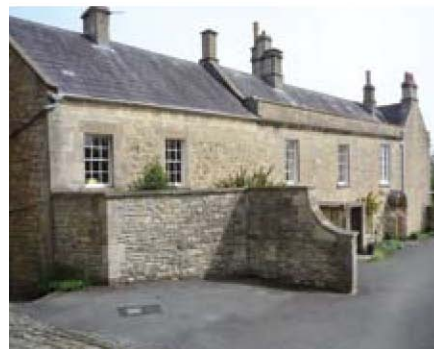
The buildings are typically constructed in local Oolitic limestone
