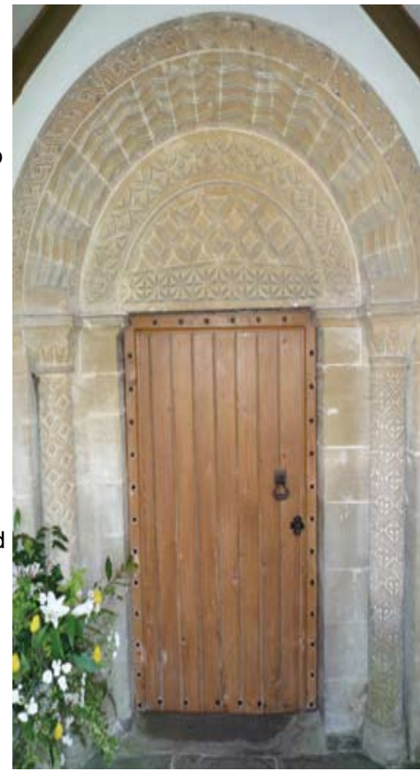
The ornate Norman north doorway to the Church of St James
