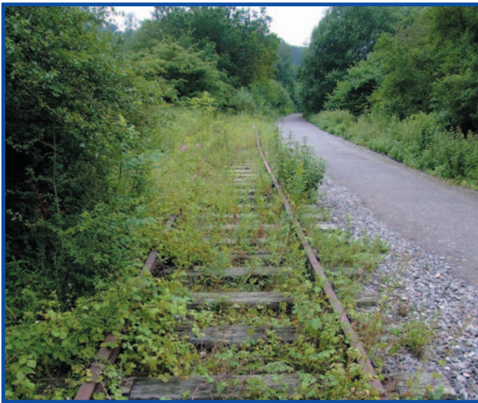
Above: Disused railway lines can provide important corridors for wildlife
