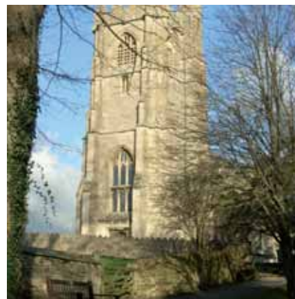
Wellow Conservation Area
