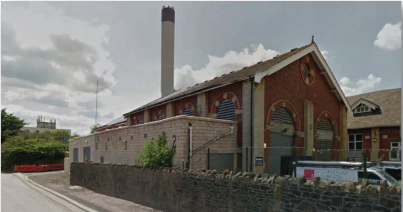
THE ENERGY CENTRE AT CREST'S BATH RIVERSIDE DEVELOPMENT, WHICH CONTAINS THE GAS CHP AND BIOMASS ENGINES WHICH SUPPLY HEAT TO THE DEVELOPMENT THROUGH A NETWORK OF PIPES. THE HEAT NETWORK IS OWNED AND OPERATED BY EON. IMAGE CREDIT: TRANSITION BATH
