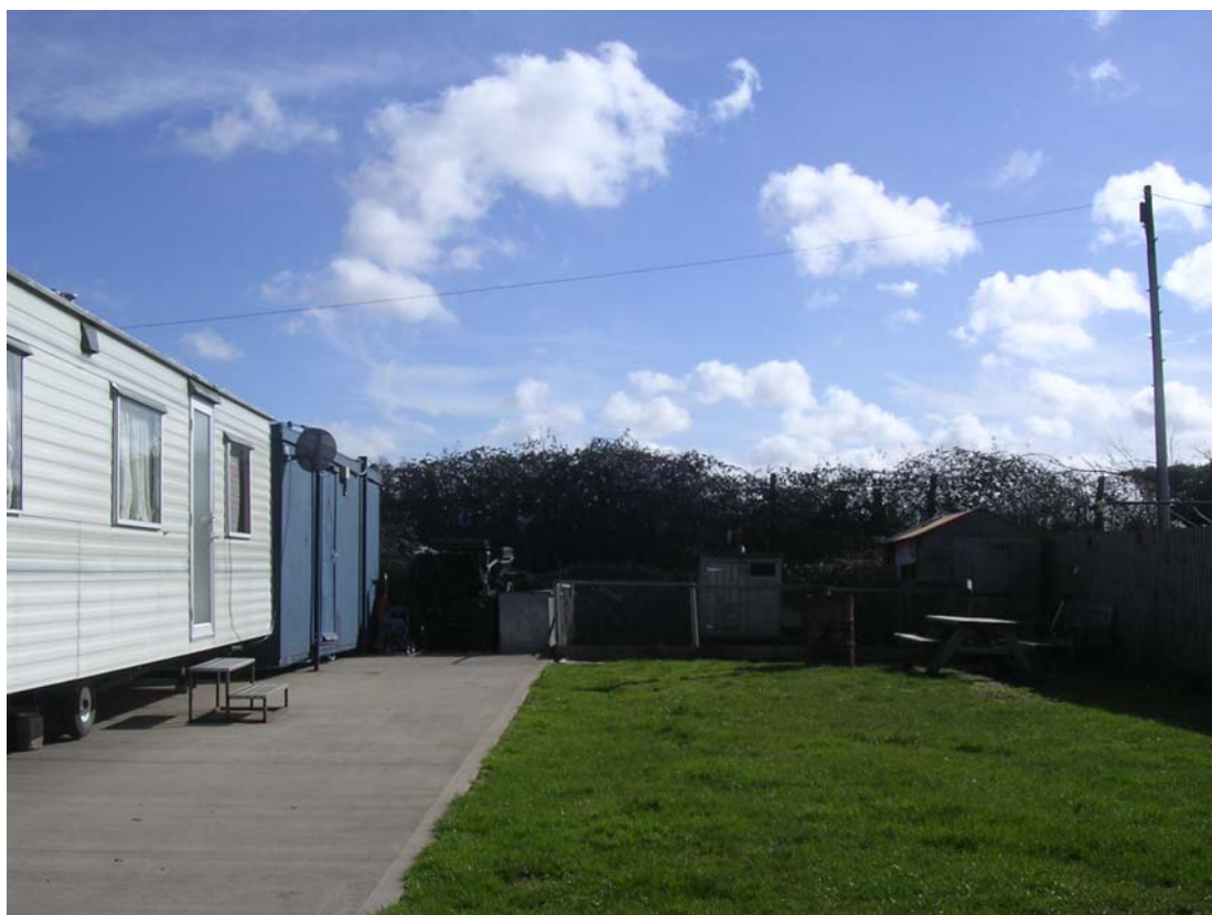
Plate 13: Large pitch on public site in South Gloucestershire
