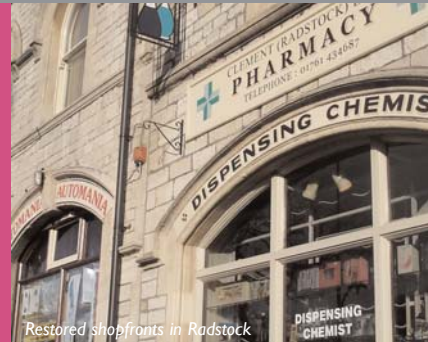
Restored shopfronts in Radstock
