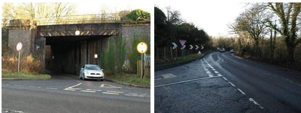
Photo 9.1 Restricted View through Bridge Photo 9.2 Poor Visibility to the Left
