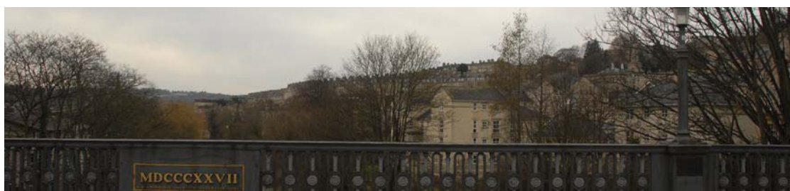
POC04 Cleveland Bridge
