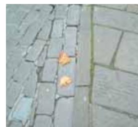
Pennant Setts, Kerb and Paving
