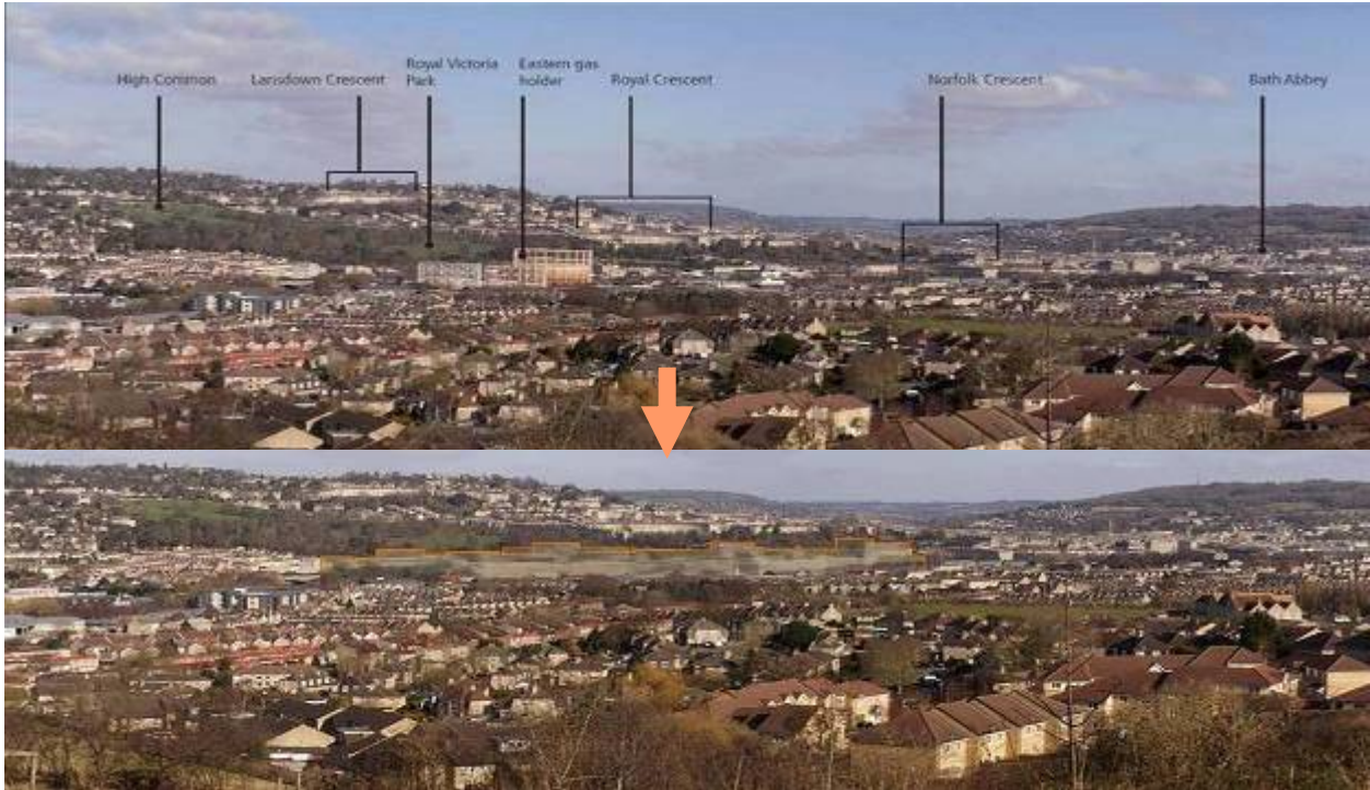
View to the City of Bath before (top) and after (bottom) the Bath Western Riverside development (picture courtesy B&NES Council)
