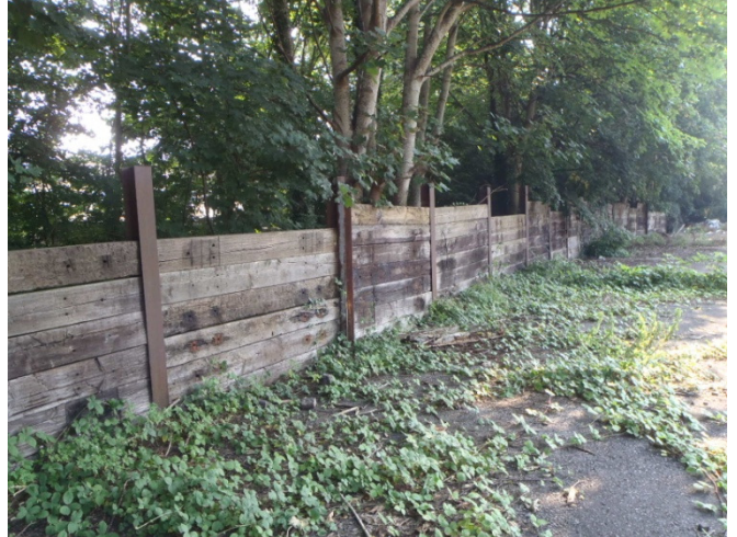
Photo 2 – RSJ and railway sleeper fence
