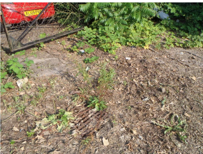
Photo 5 – Surface water gully by access gate.
