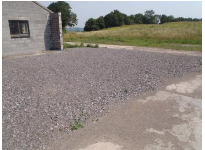
Photo 10 – Capped mine shaft with Building 3 behind
