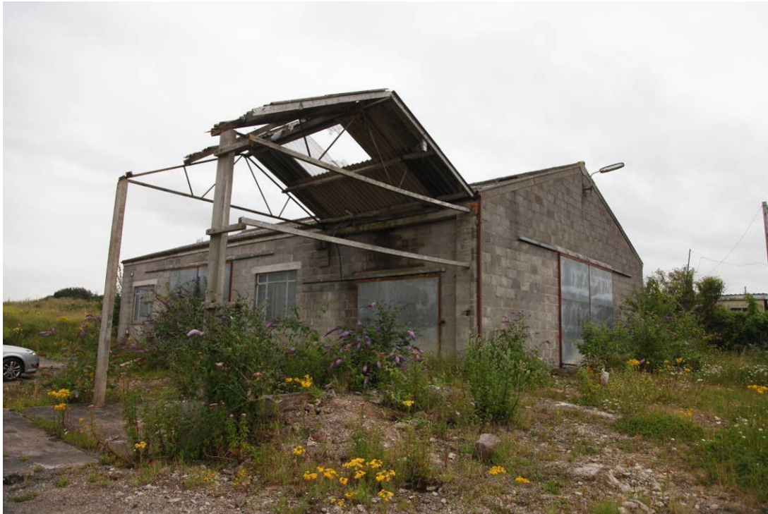
Plate 3: Building 2 viewed from south-west
