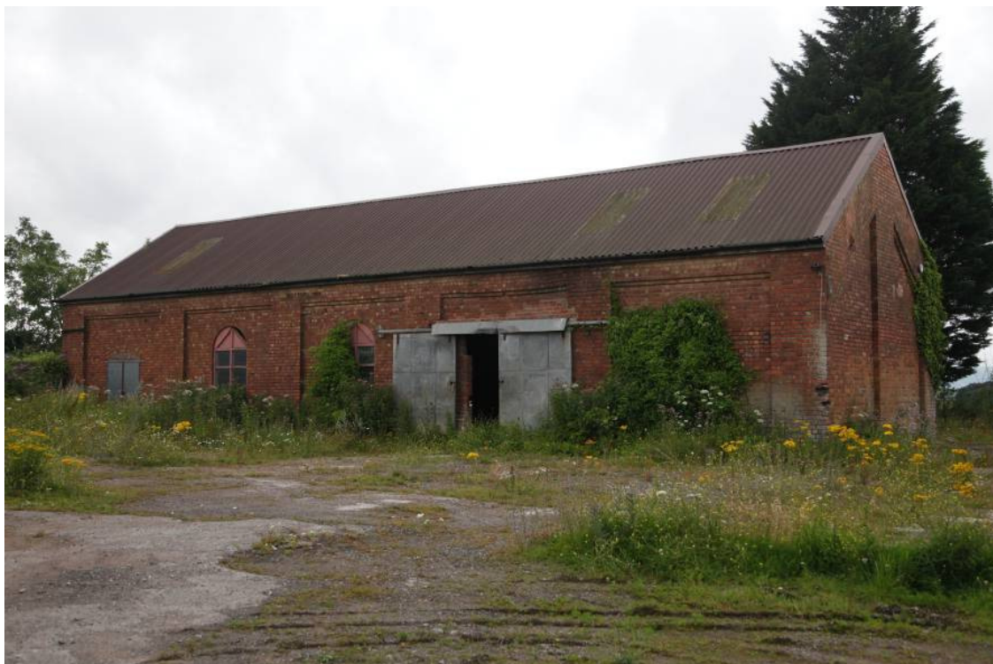
Plate 1: Building 1 viewed from east
