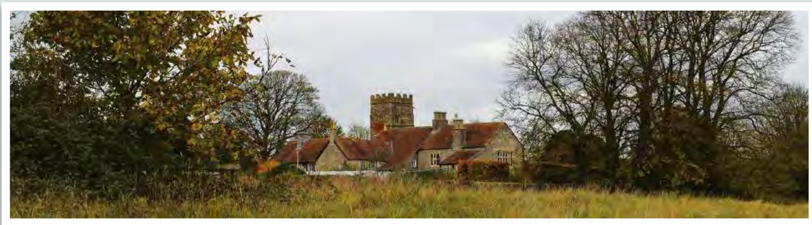
Church Farm House & Ruins of St. Helen's Church/Old Church of St. Helen – looking north west.
