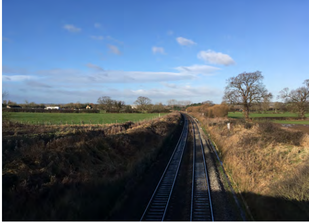
VIEW ALONG GREAT WESTERN MAIN LINE
