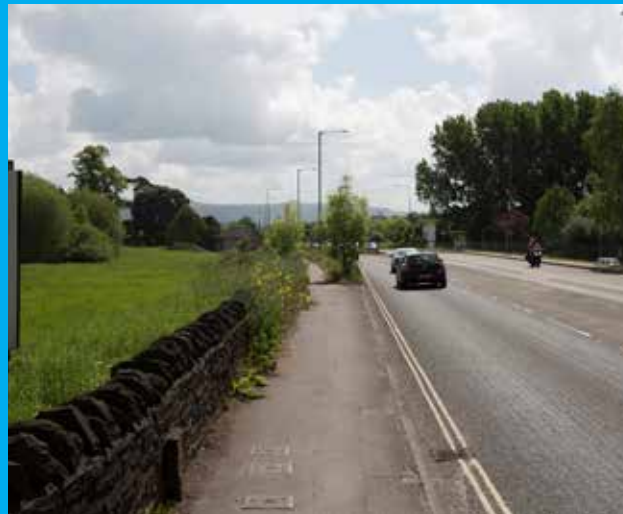
View east along the A4 towards Hicks Gate roundabout
