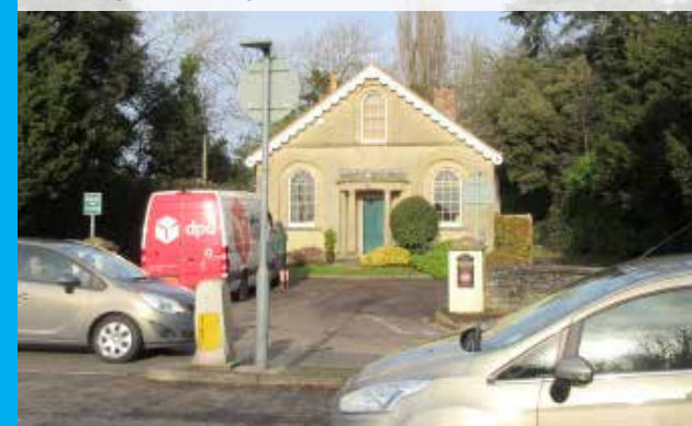
The lodge to Brislington House
