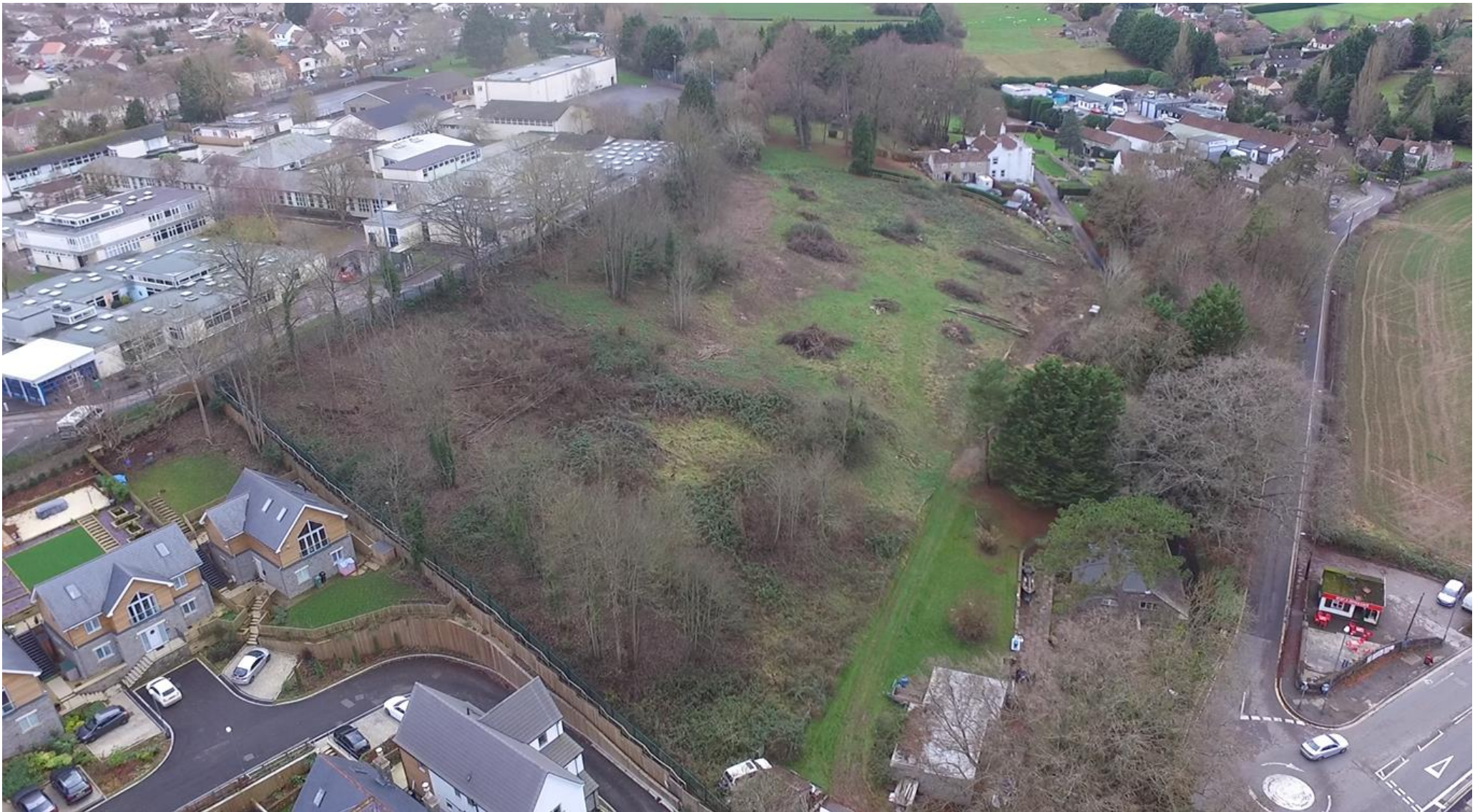
Photo 4. December 2018 drone view of the site which also shows the new Treetops residential development to the east of the site. Any development of the site would retain / replace the existing trees on the southern boundary of the site to maintain the existing screen of the existing Broadlands Academy school buildings, which are only visible during winter months.
