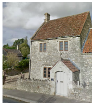
PHOTO 9: Stone Walls and Porches are key features
