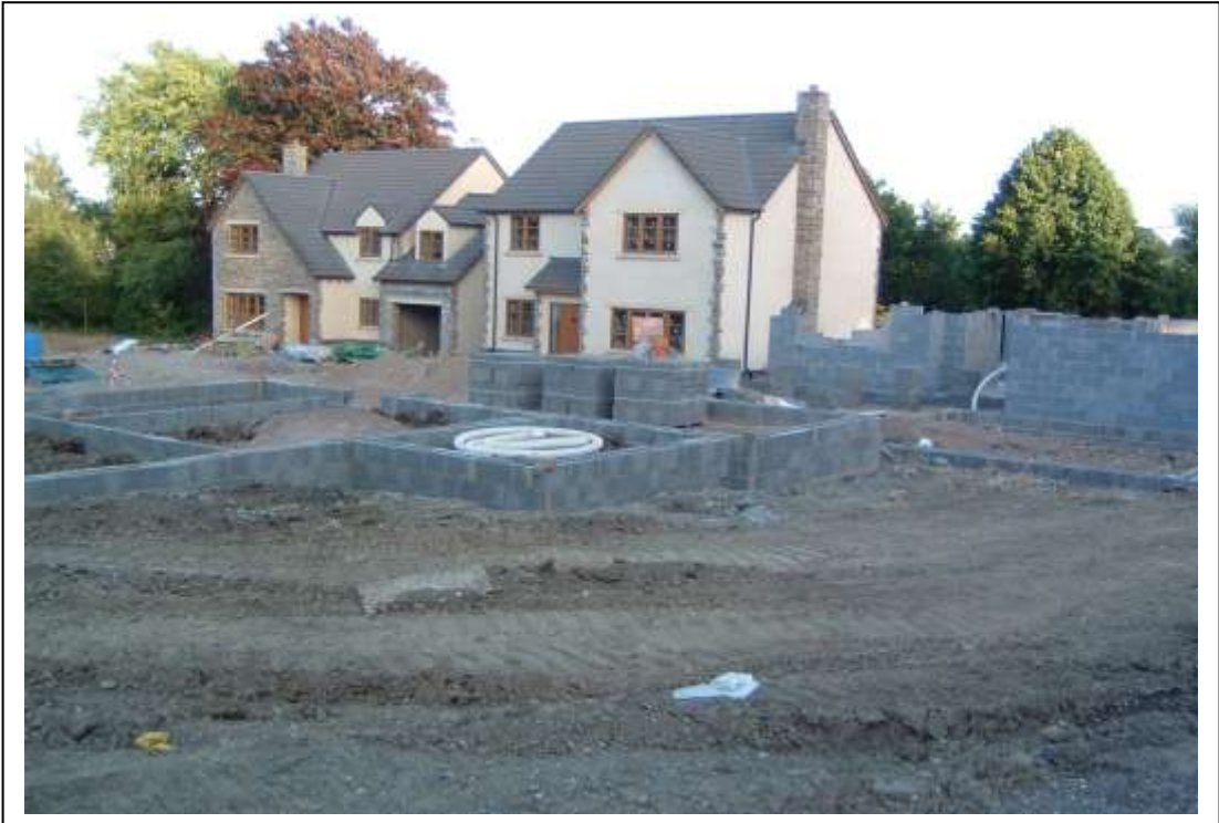
Housing Development at The Sidings under construction
