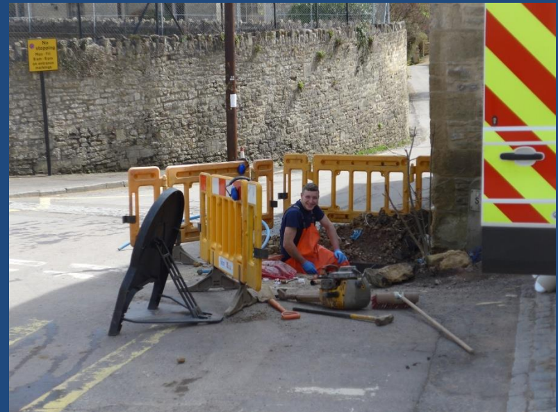
Cobbles at each 'entry point' and junction (Wellow)
