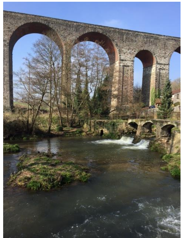
3 – Pensford Viaduct and the Weir
