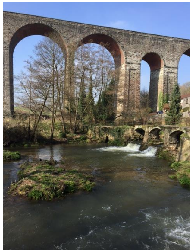
3 – Pensford Viaduct and the Weir
