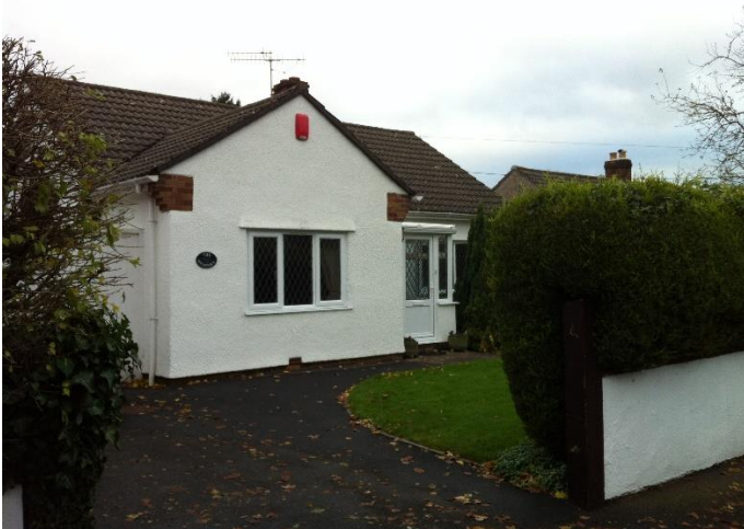
Picture 9 Rendered finish, roman roof tiles
