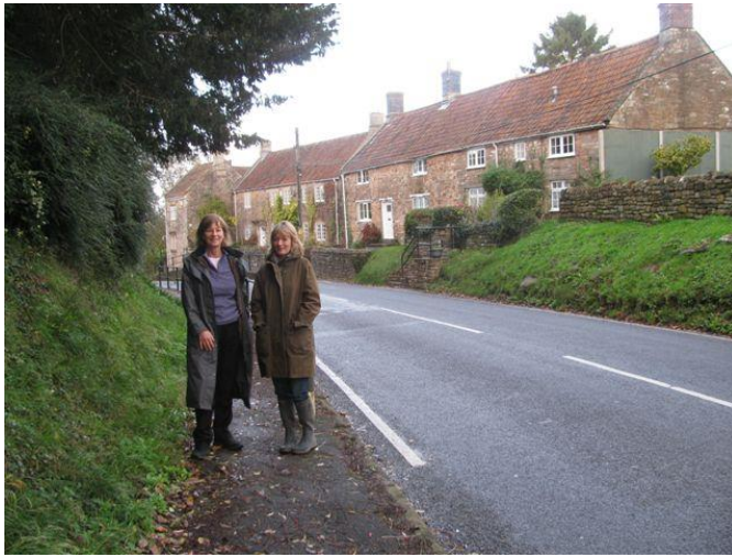
Picture 40 Stowey showing older terraced cottages, built in local stone, with clay roman roof tiles & survey team
