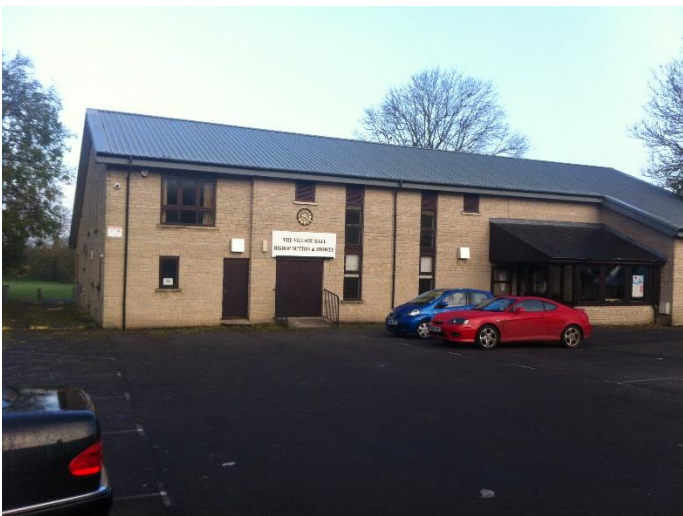
Picture 33 Village Hall on Wick Rd
