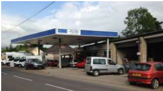
Figure 11 F E Brent and Sons Garage
