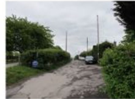
3. Access roads to businesses
