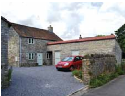
Greenway Cottage (Front)
