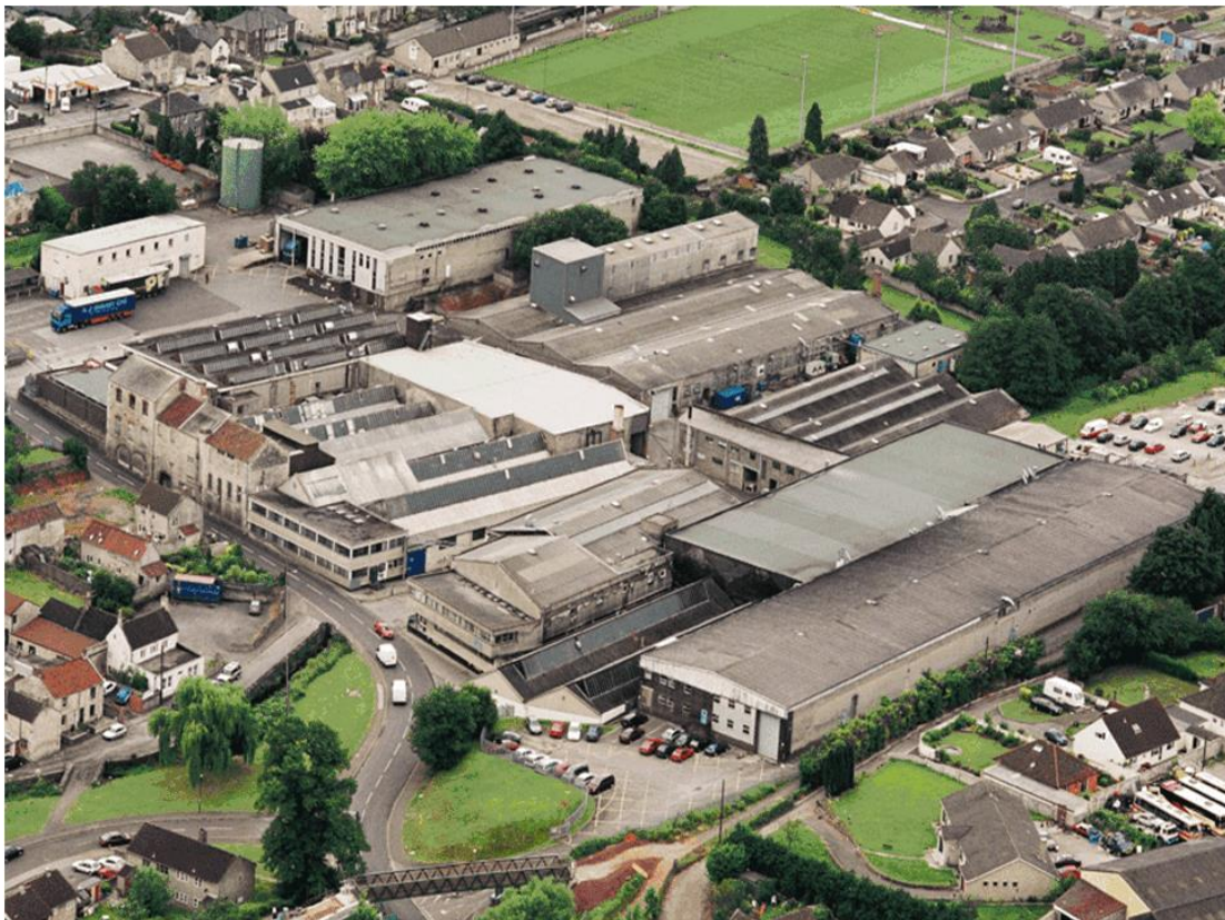
Aerial view of FWMS Site SSV 4, Vol 4 Somer Valley
