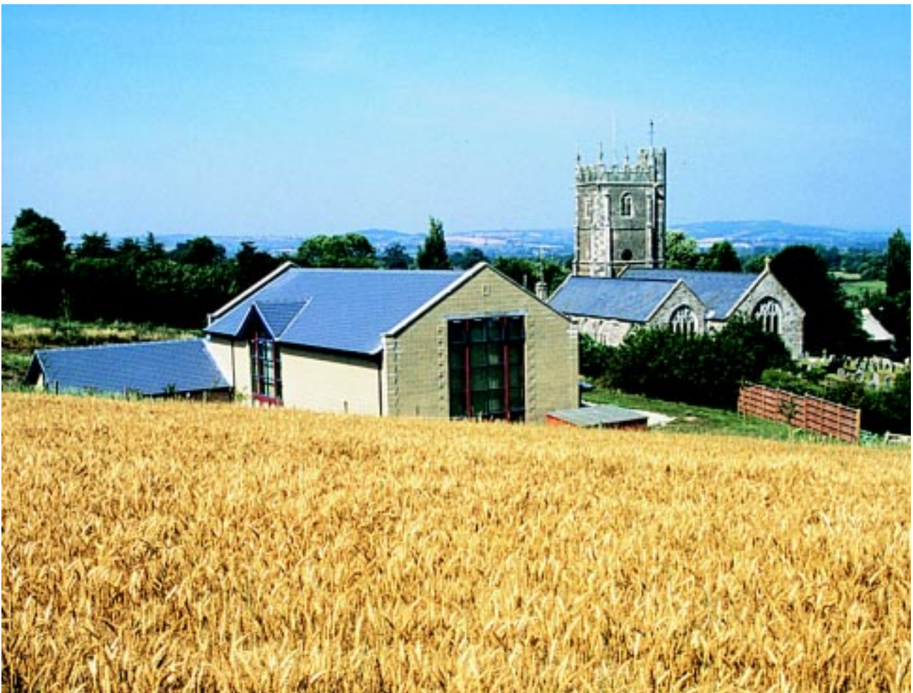
New development in villages can be both compatible with local character and modern, while meeting village needs, as in this new village hall in Kentisbeare, Devon.
