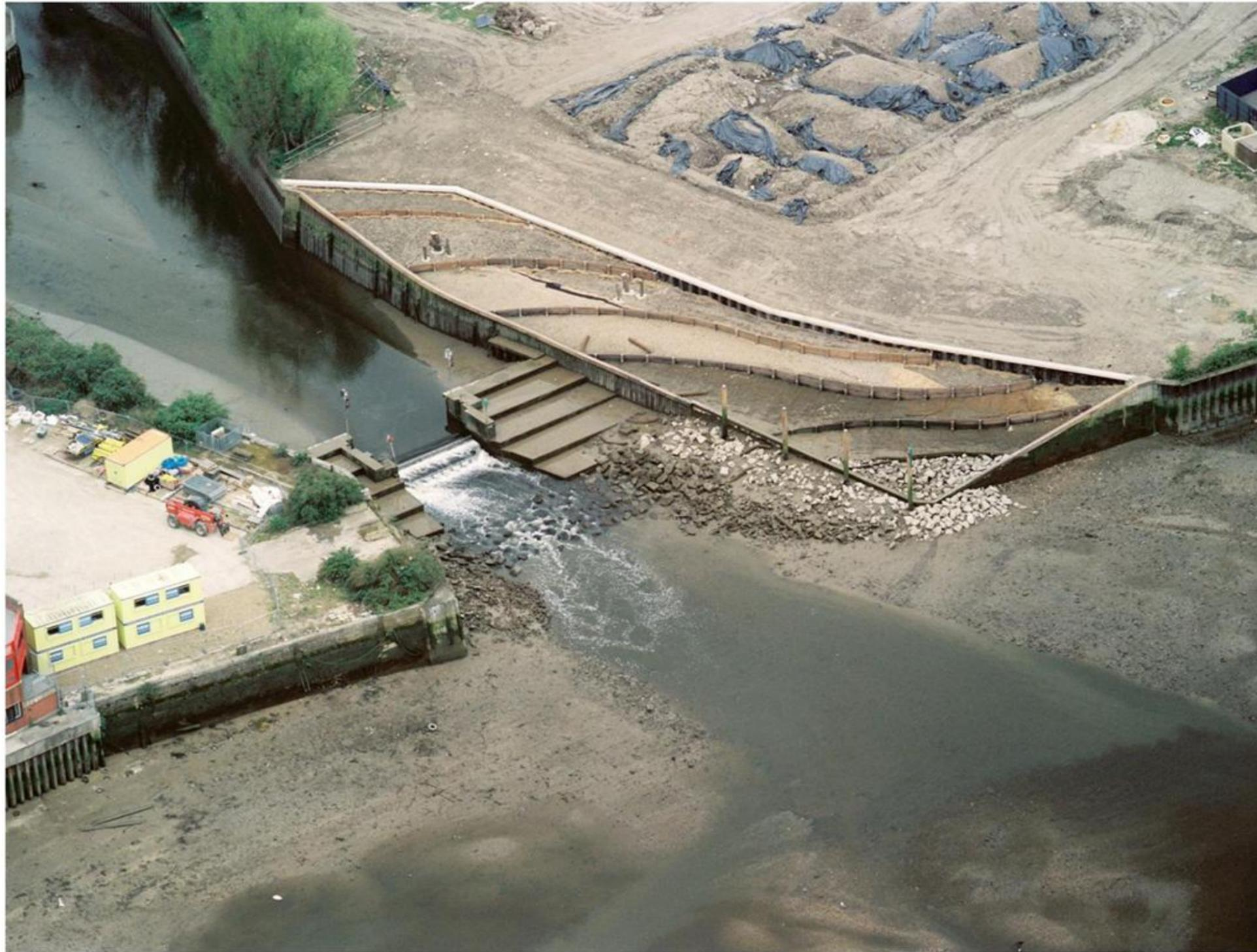
**Plate 7.6:** Stabilisation of substrate on new terraces with coir matting and rolls, River Wandle, London
