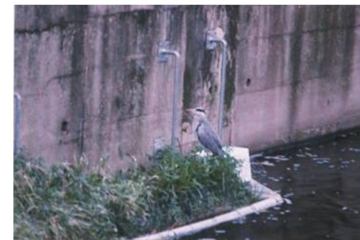
Figure 7.4: Inset planters/vertical beaches on sheet piling
