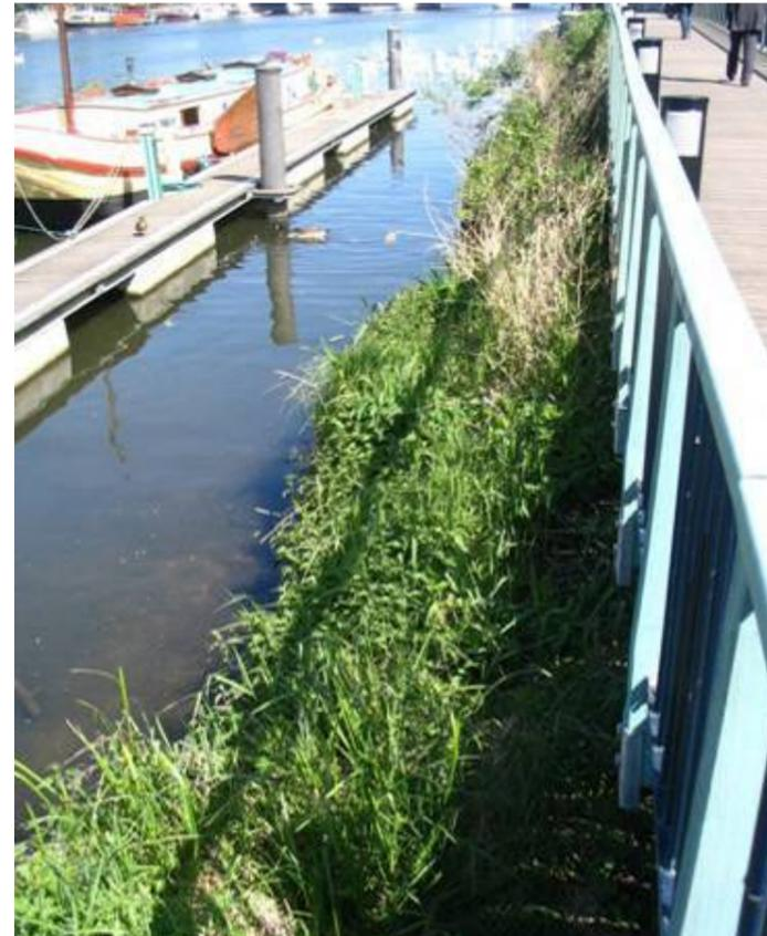
Plate 7.10a & b: Vegetated rafts on fixed guide rails, Charter Key, Hogsmill River
