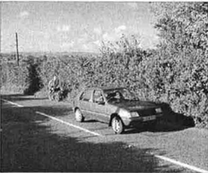
A39 at Hallatrow Hill - speeding traffic and no pavements
