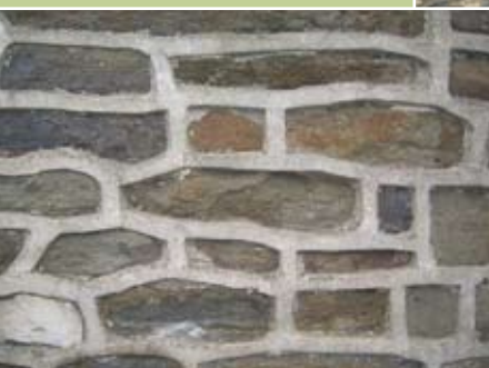
Inappropriate pointing can permanently damage stone walls
