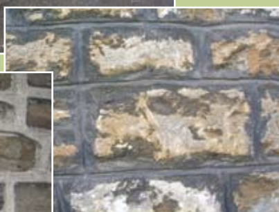
Inappropriate pointing can permanently damage stone walls
