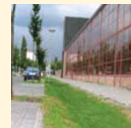
create swales to hold the rainwater
