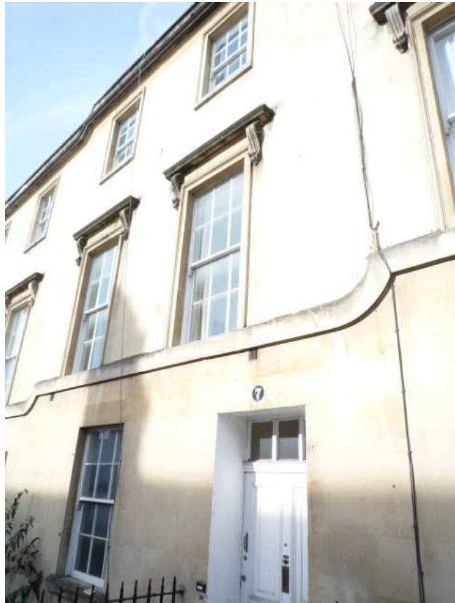
E) Refurbishment and extension of a Grade II listed building incorporating energy conservation measures (7 Charlotte Street; view application)
