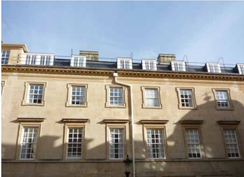
A) New slim-profile double-glazed windows in Grade I listed building (St John's Hospital, Bath City Centre; view application)
