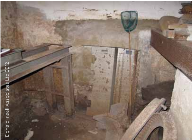
Donald Insall Associates Ltd 2012
