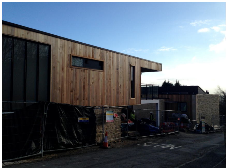
Image 5: Side view of interpretation centre, partial completion. Jan 2014.
