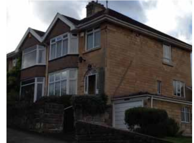
Example of an Early 20th Century Building in Bath & North East Somerset
