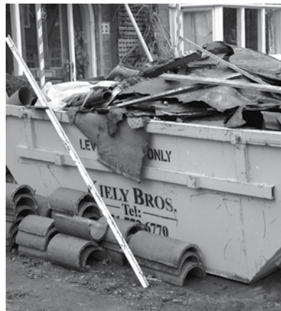
Segregating waste onsite for recycling
