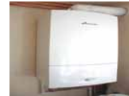
gas condensing boiler
