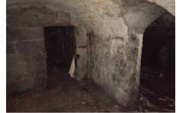
Series of interconnected vaults beneath Milsom Street
