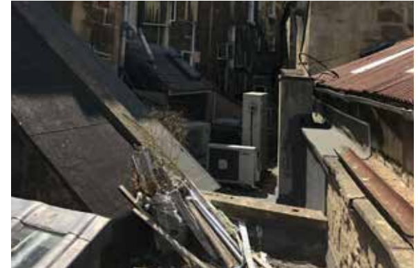
Series of flat roofs to the rear of New Bond Street
