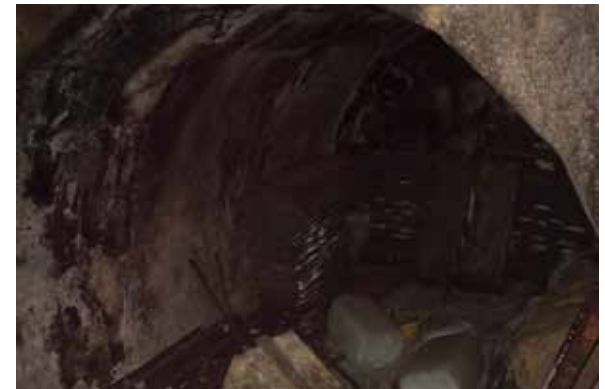
Un-used vault beneath New Bond Street
