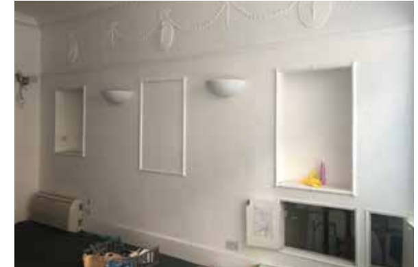
29 Milsom Street; Contemporary interior lining
