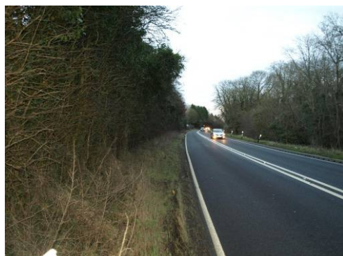
Photo 4.1 Access Position: View South
