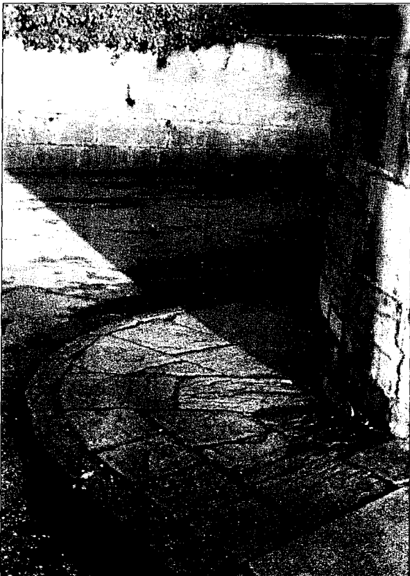
Traditional pennant stone paving
