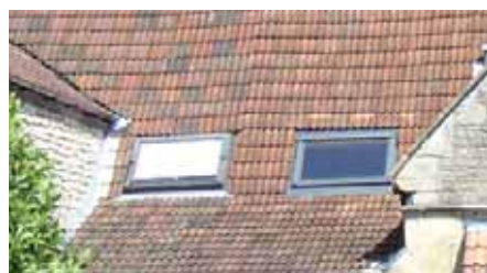
Modern rooflights can detract from the historic character of buildings
