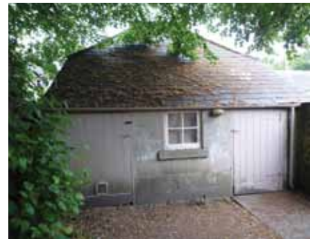
Combe Hay Manor Gas House
