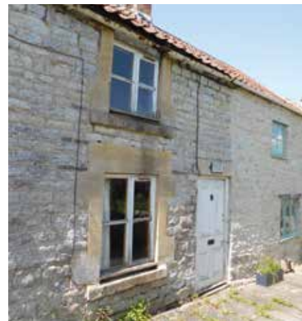
No 2 The Batch – currently being restored
