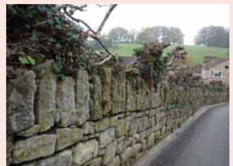
Traditional walling is an important feature and common boundary treatment
