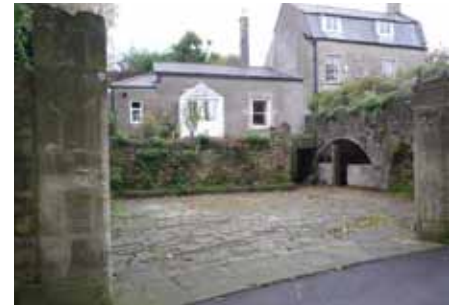
The locally important buildings make a significant and positive contribution to the character of the Conservation Area
