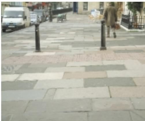
Poor visual quality of patchwork concrete paving Good quality workmanship
