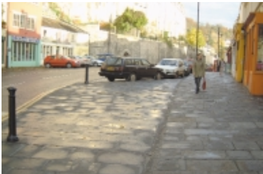
Pavement widening using reclaimed pennant
