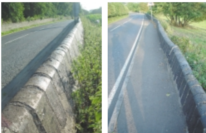
Moulded coping stones on walls in Corston and Kelston
