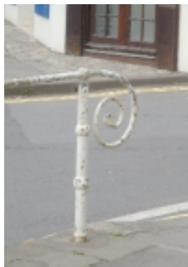
Locally distinctive ironwork in Chew Magna
