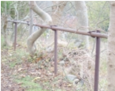
'Temporary' railings outside Keynsham Hospital
