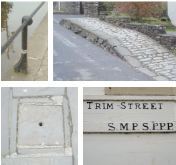
Clockwise: Post and railings made by the William Evans Foundary. Historic paving in Pensford. Incised street lettering. Pennant coal hole cover.
