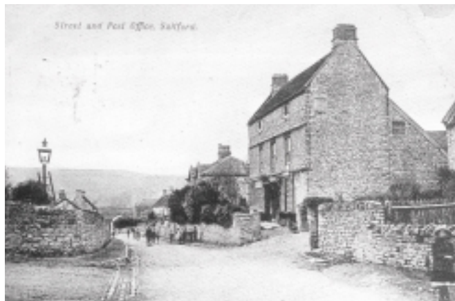
Street and post office, Salford
