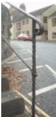
Iron railing detail, Weston
