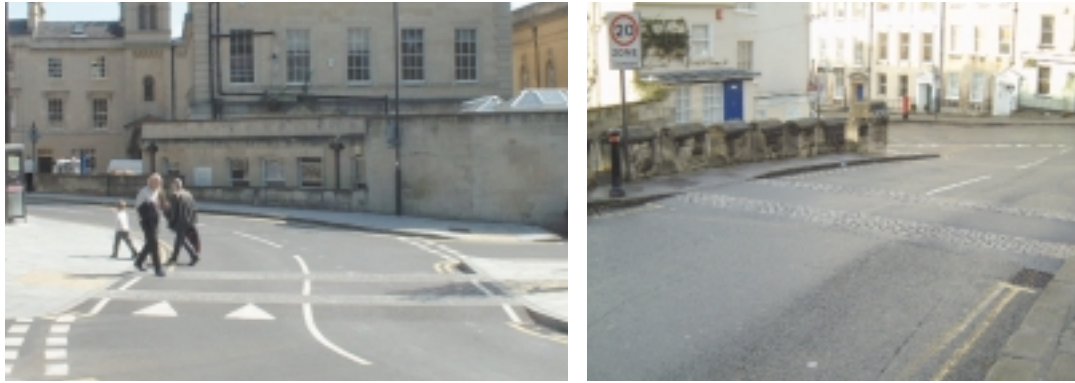
Sensitively designed pedestrian crossings at Charlotte Street car park and Camden Crescent.
