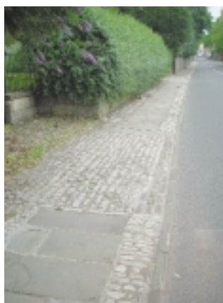
Left: Pitched setts at Newton St. Loe
